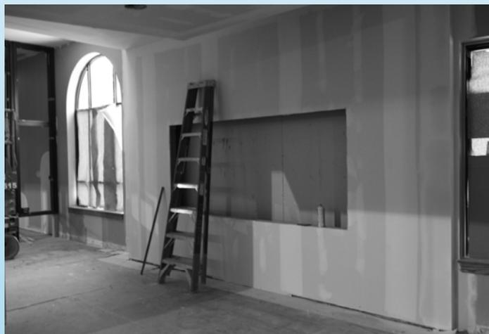
New cabinetry is being installed along the North wall of the sacristy where the sinks were. Much of the drywall has been taped and sanded; the windows frames along Armitage Avenue await stained glass; the reredos panels, a decorative screen behind the altar, have arrived; dark wood paneling is being installed; to the right is a niche for an icon.
