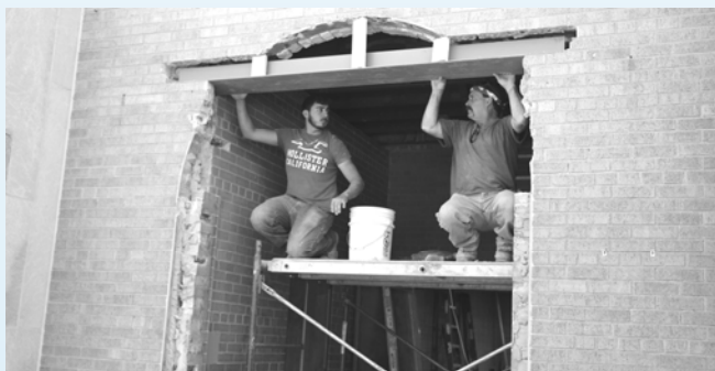
Lintel being installed on Armitage Avenue doorway
